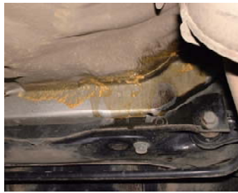
Rust proofing agent applied to joints, panels, welded spots etc.
