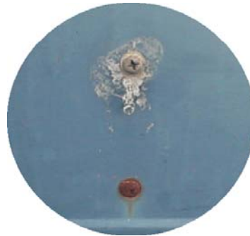
2 year bolt exposure test result: Top bolt was treated with Noxudol rustproofing agent. Bottom bolt was not treated and as a result it rusted.
