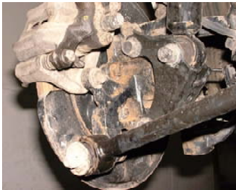
Apply rust proofing agent to bolts, nuts etc. Any parts that shows Signs or rust or exposed to rust.
